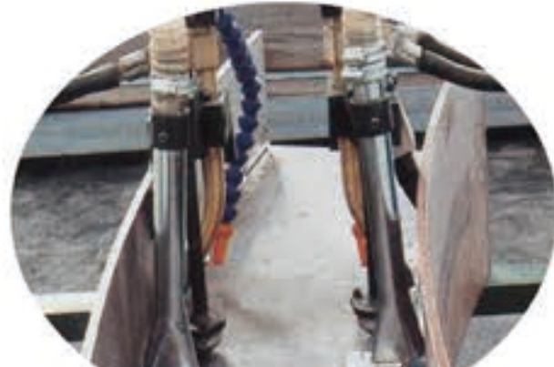
腹板H型钢的焊接 Welding of the Rib of the H-beam
